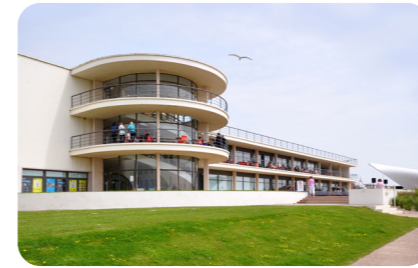
De La Warr Pavilion, England
